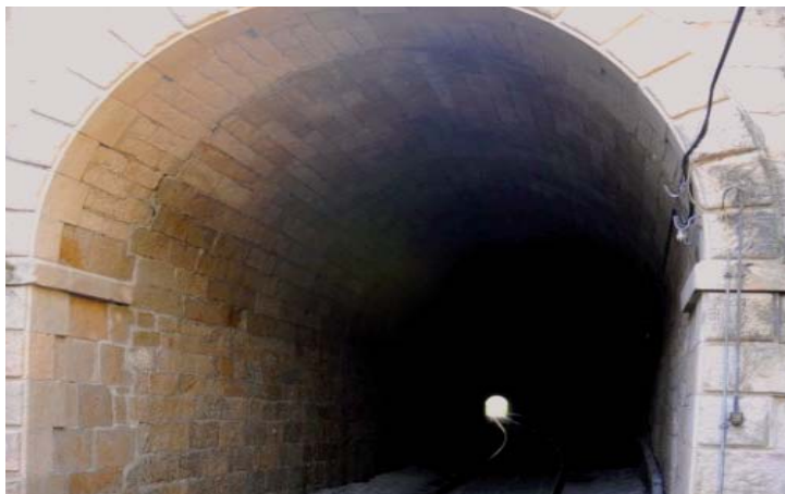
Image 2: The first railroad tunnel already cleaned with torbo
