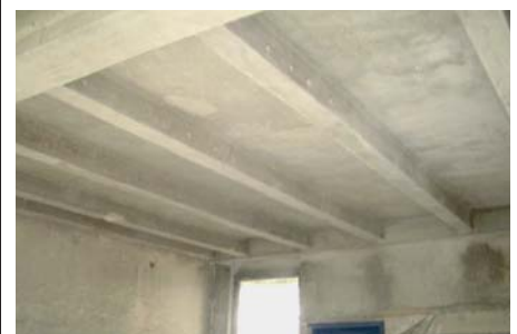
Image. 5: building Kistlerhofstraße, Munich
