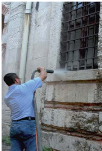
Image 2: cleaning the facade
