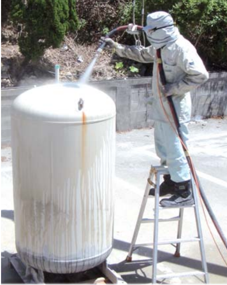
Image 6: removal from rust at tanks
