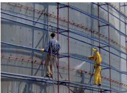
Image 2: torbo blasting at the tank
