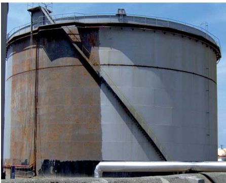
Image 1: oil tank before / after
