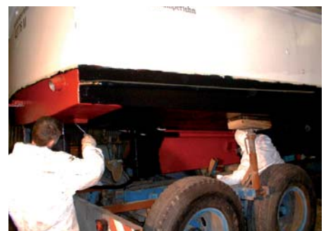
Image 6: put on the new coating
