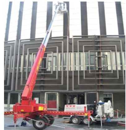
Image 12: Renovation with the man lift and the torbocar AC37
