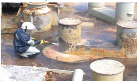
Image 9: removal of rust with torbo
