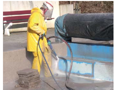
Image 3: Working with torbo and UHP unit
