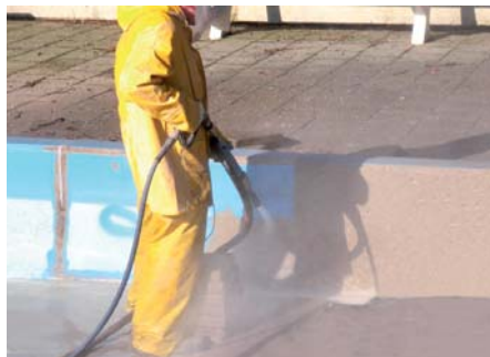
Image 2: removal of polyester coating with the torbojet-system
