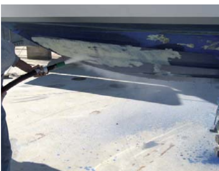
Image 4: Removal of antifouling
