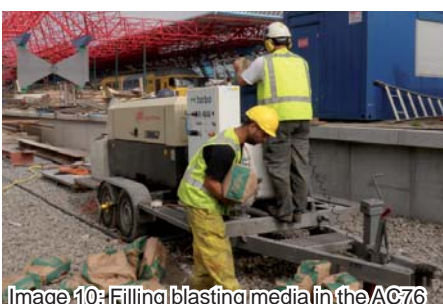
Image 10: Filling blasting media in the AC76
